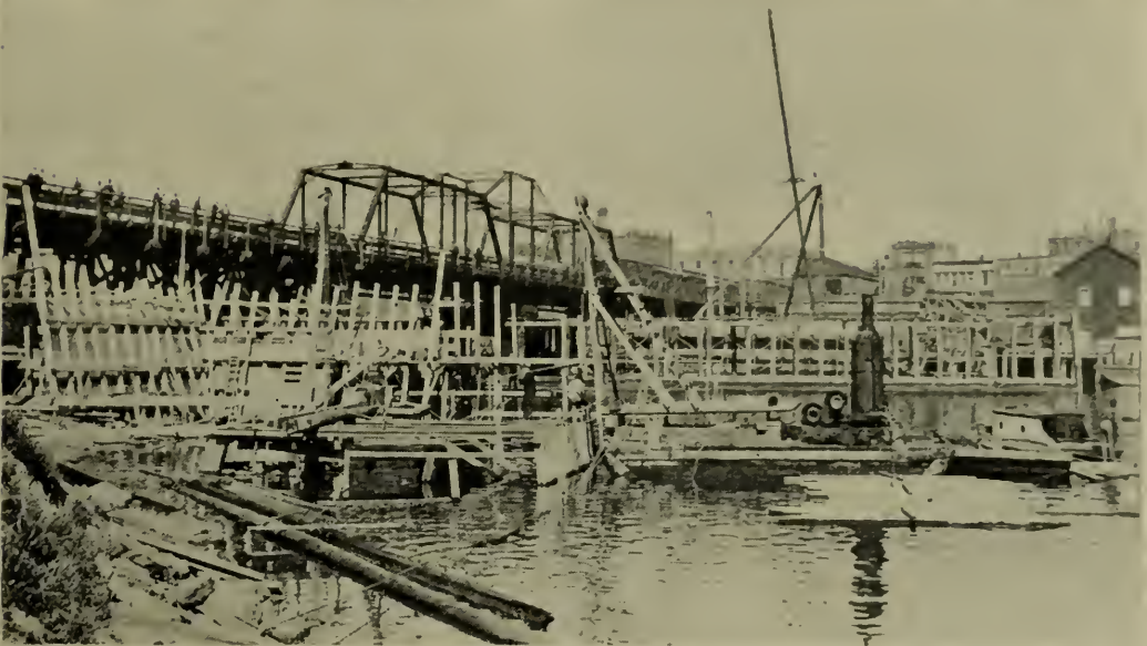
FIG. 9. GENERAL VIEW FROM WEST.
